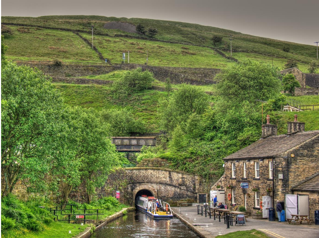
Standedge Tunnel, Huddersfield Narrow Canal © 54north
